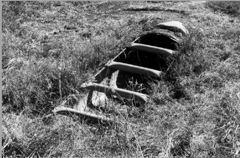
FIGURE 3.12 Safety treatment for parallel drainage pipe
