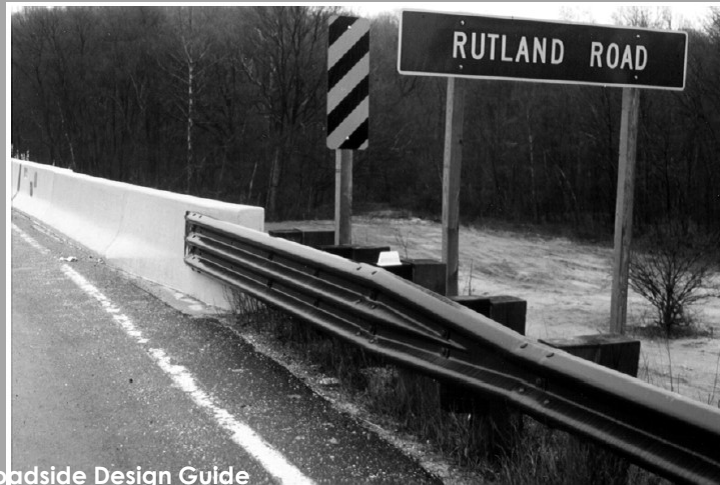
FIGURE 7.19 Thrie-beam transition to modified concrete safety shape
