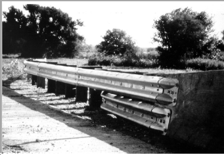
FIGURE 7-17. W-beam transition to vertical concrete rail
